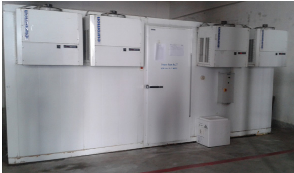
Figure 20. Freezer Room 50 m 3 Capacity at Store
