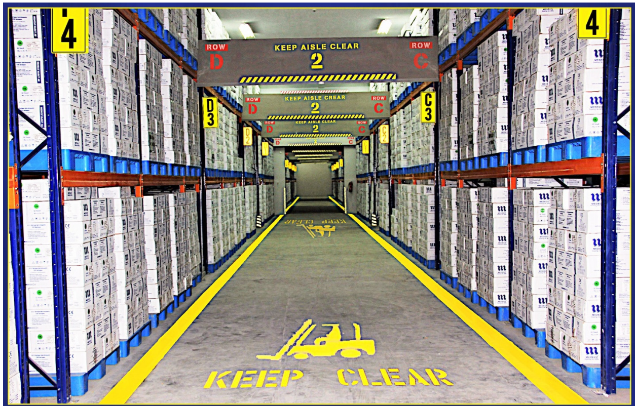
Figure 40. Pallet Racking System at Warehouse
